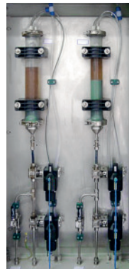
Settlers installed on-site for some of our process analyzers in pulp and paper mills.
